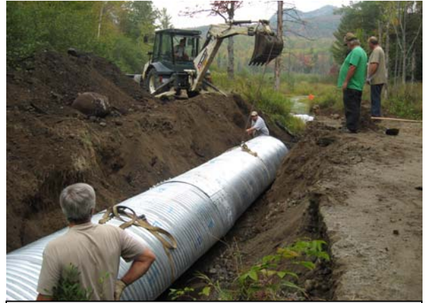
Town of Chester highway department installing a new culvert to improve both public safety and trout migration in the stream system
