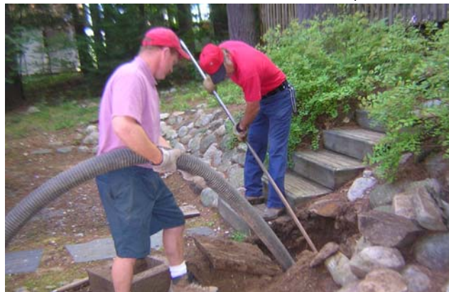
Septic hauler pumping out a residential septic tank
