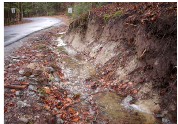
Eroding clay road ditch on Adirondack Road
