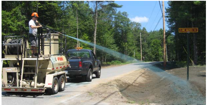
Warren County SWCD staff "hydroseeding" a bare road ditch to stabilize it. The mix of seed, water and mulch will rapidly establish a new grass sod in the ditch, controlling erosion.
