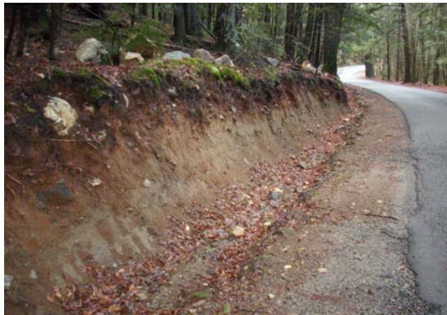
A section of Hoffman Road where the ditch was recently excavated to maintain drainage capacity. This ditch is showing signs of erosion and sedimentation.
