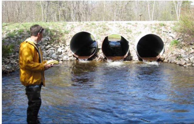
Stream culverts on Adirondack Park Road on Rogers Brook, which are a barrier to fish passage because they are higher than the stream.
